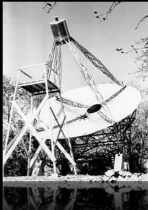
Reber's Radio Telescope, 1937
