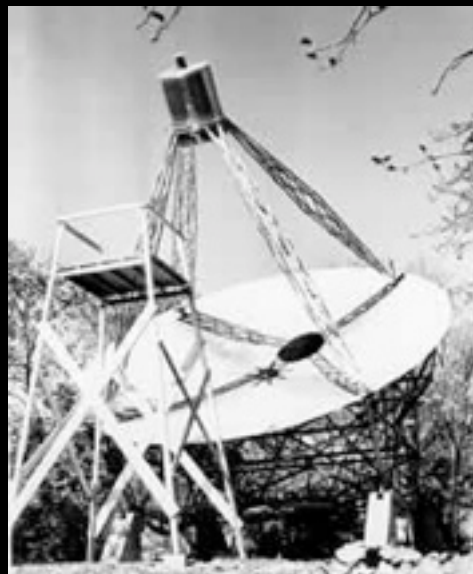
Reber's Radio Telescope, 1937
